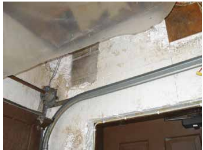
Exposed foam insulation in garage should be removed or covered
