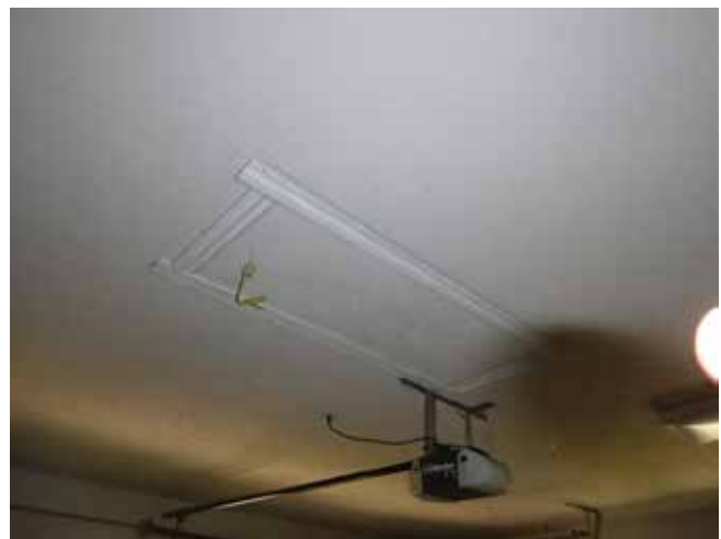
Non-rated pull-down installed in garage with drywall laminated to cover
