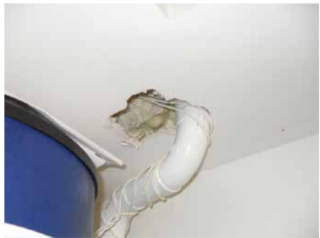
Garage ceiling penetrated by central vacuum system.
